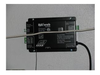
The Control Module is mounted near the furnace where the thermostat cable is routed.
