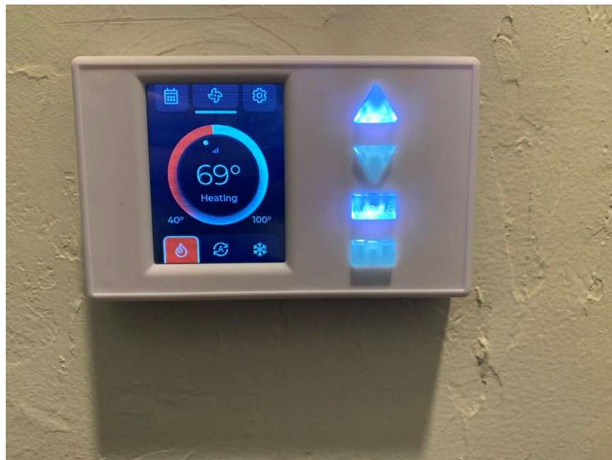
Test each function, Heat, Cool and Fan by tapping the mode buttons. You can also test the Auto mode by tapping the Auto button in the center.
